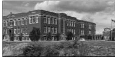
The newly renovated Marblehead Veterans Middle School
